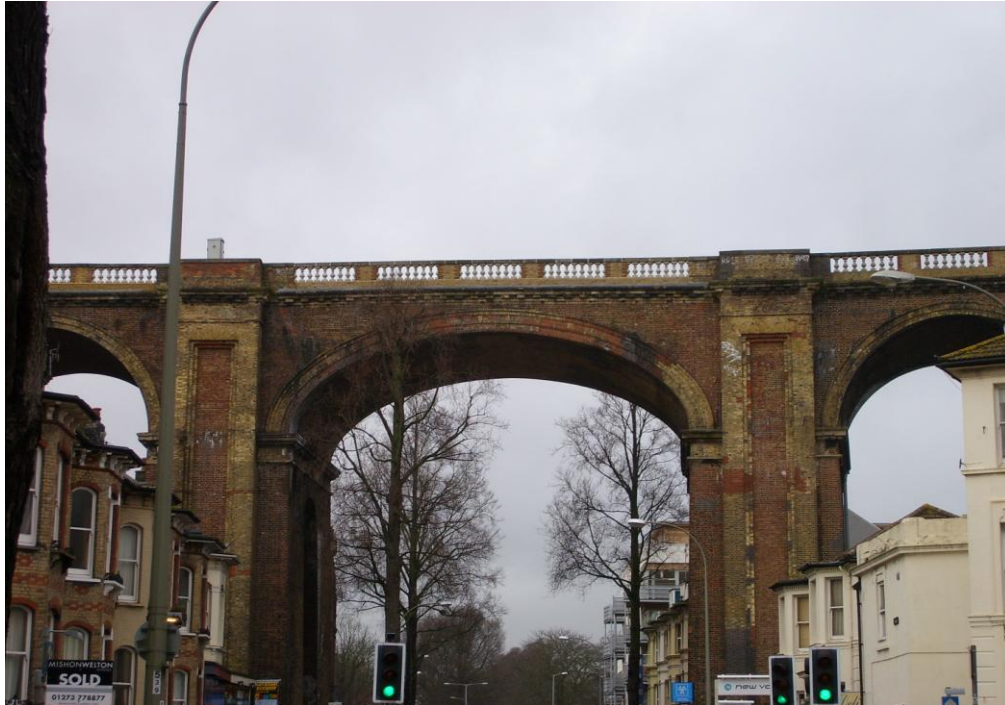
[Figure 5.1 shows a typical train bridge viaduct in Brighton, UK]
